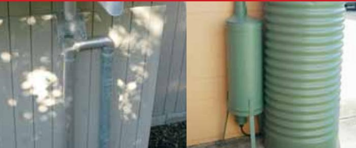
(Above) A galvanised steel stand is an optional alternative to post or wall mounting.
