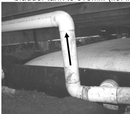
**Not Recommended:** Over flowing water should not have to rise vertically before overflowing
